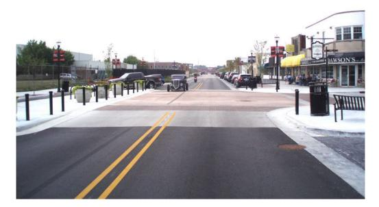
Another approach is to elevate crosswalks to act as a speed hump. This can either be done at a crosswalk, or across an entire intersection. The longer configuration of the raised area covering the entire crosswalk is better for emergency vehicles which can navigate the longer surface change at a better speed. This approach would require each intersection to be reconstructed to provide a distinct bump as people drive through the corridor.
